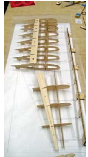
Wing construction under way with FLE tacked to the building board with pinning tabs and the ribs in place on SW-A, SWB and SWD will be installed next.
